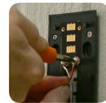
The wiring must be connected to a transformer with a voltage of 8VAC - 24VAC and an internal doorbell or resistor.
