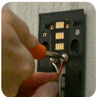
**i** The wiring must be connected to a transformer with a voltage of **8VAC – 24VAC** and an internal doorbell or resistor.
